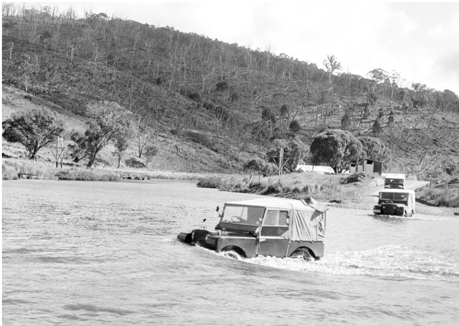
Landrovers crossing the Eucumbene River near Adaminaby Portal site camp. Photo from National Archives of Australia: A11016, 497. Barcode 4240556
