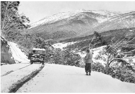
The Alpine Way under construction. Photo source unknown.
